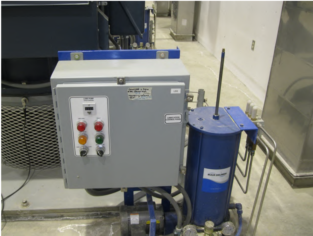
Figure 16-1. Automatic Grease Lubrication System for a Vertical Pump.
