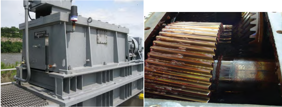
Figure 16-7. Gear Reducer for Miter Gate Drive.
