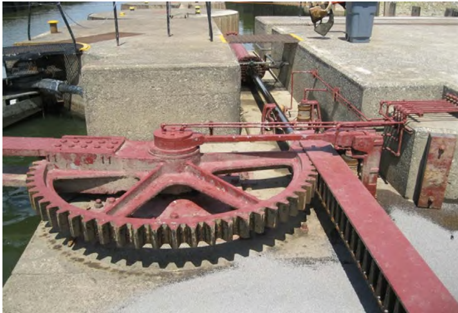
Figure 14-3. Sector Gear and Rack (Rack and Pinion).
